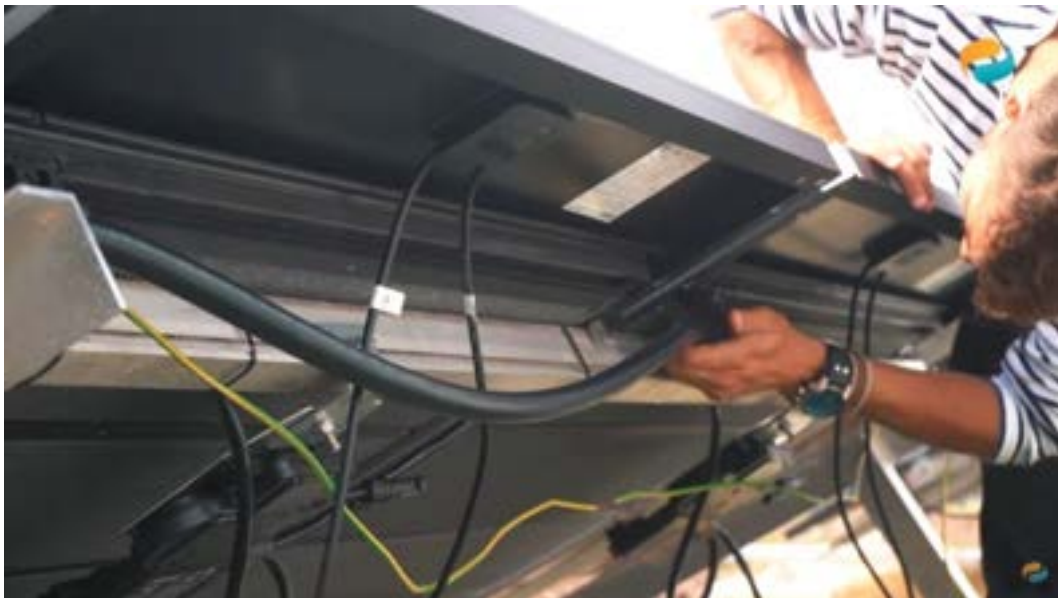
Figure 23: DualQuickfit coupling simply need to be clipped on to be leaktight
