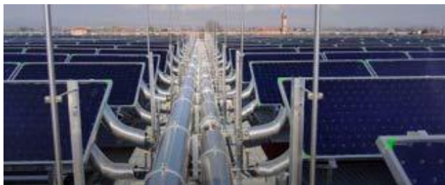
Figure 1: HVFP-based system for industrial process heat (hot water & steam) in Turin, northern Italy
