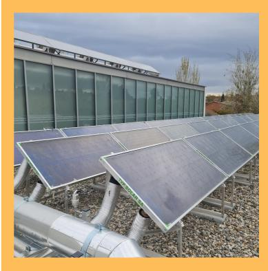
The TP3 system is integrated with the existing HVAC system, incorporating the TVP panel, the Fahrenheit hybrid adsorption chiller, and the RatioTherm stratified tank. The new system is connected in series upstream of the existing heat pump.
